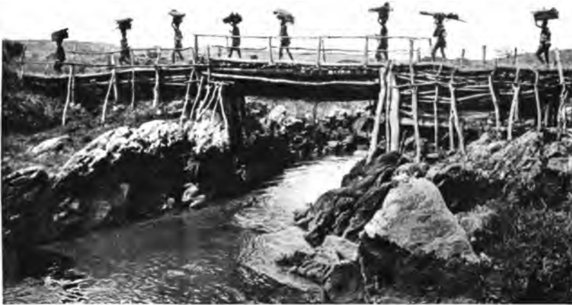
A BRIDGE ON THE HIGHWAY
